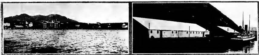
The White Pass & Yukon Route hotel at Lake Atlin and the wharf at Skaguay.
